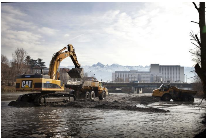
Figure 1. Extractions from a bank removal in Grenoble along the Isere river.
