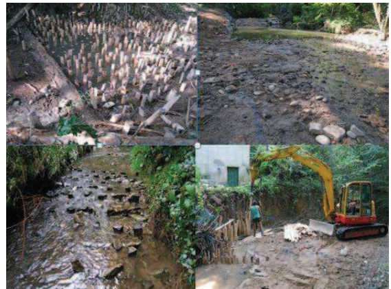
Illustrations concernant la pose de semis de piquets (dimensions fictives)
